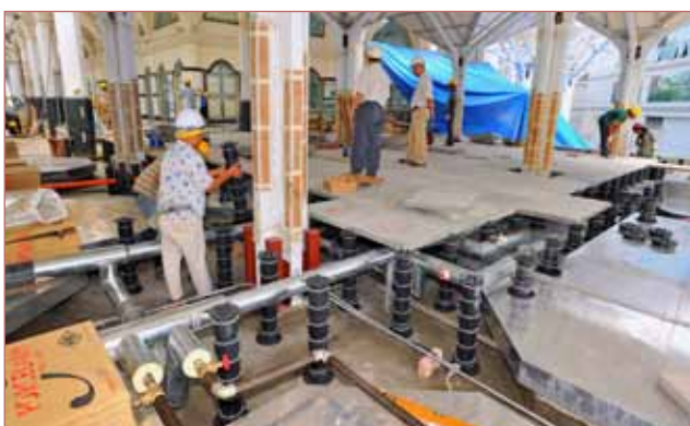
VersiJack® allows easy accessibility to services when required
