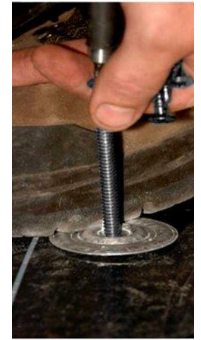
Mechanically fastened
