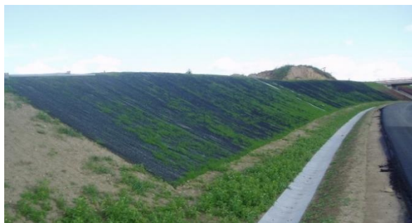
Installation of K-Mat
