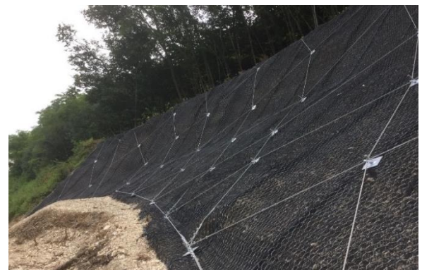
Installation of K-Mat RF Metal
