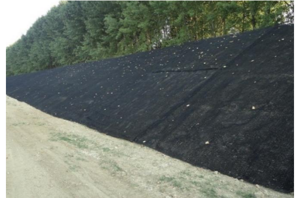
Installation of X-Grid AM
