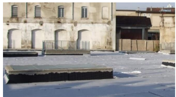
Installation of Q-Drain ZW as drainage layer in a green surface
