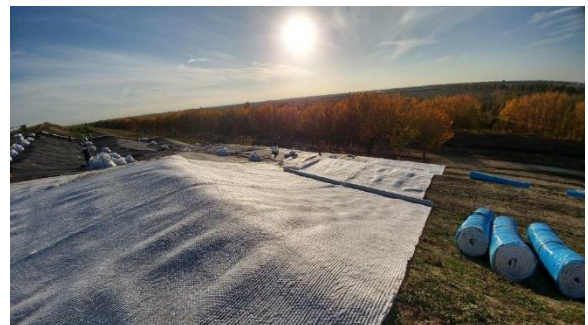
Installation of Q-Drain C as drainage layer in a landfill
