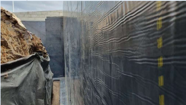
BituBOND BondSEAL Installed
