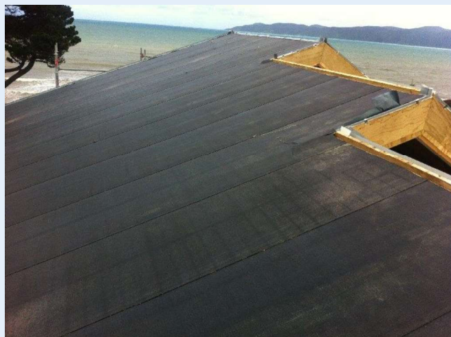
BituBOND BondSEAL installed under roofing tiles
