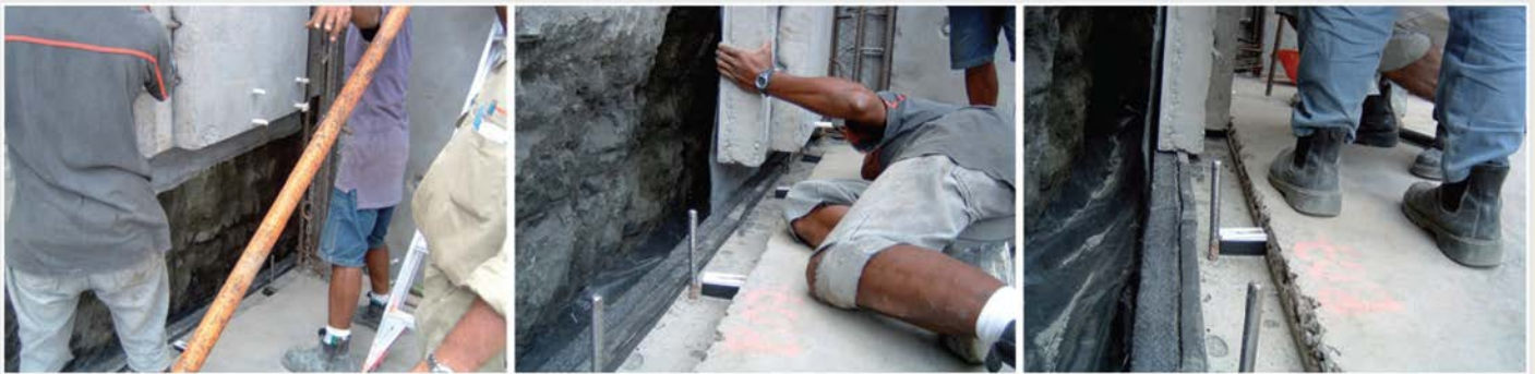
Right: MidCity Plaza, Fiji, Access behind the walls is impossible Below: in this situation the rawMAT membrane is pre-installed to the panels. Careful placement of the panel allows a watertight floor:wall junction to be formed
